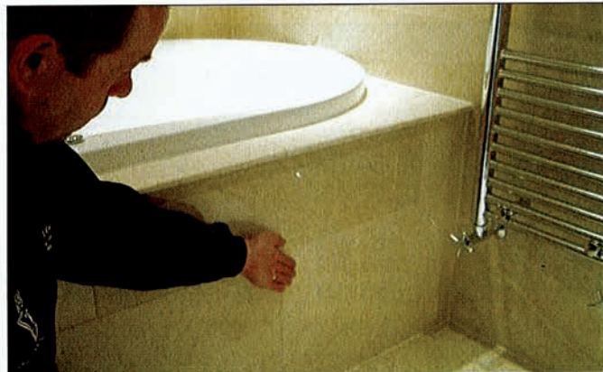
Paul Coyle shows the concealed access panel.
